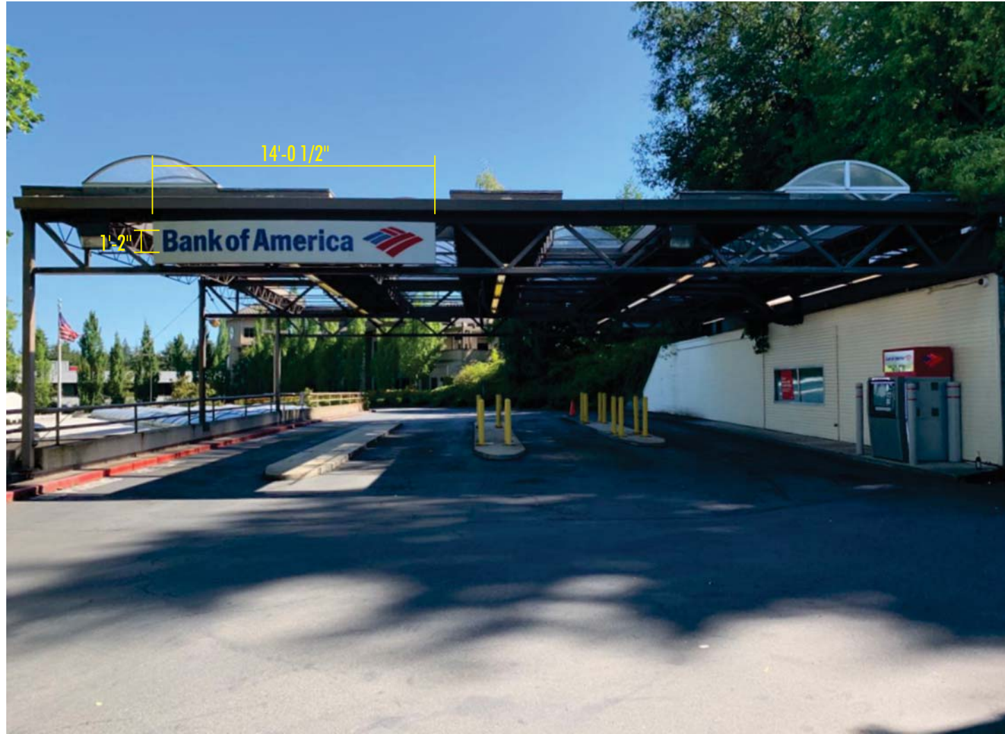
EXISTING SIGNAGE | TO BE REMOVED & DISCARDED | PATCH & PAINT HOLES T/M FASCIA COLOR
