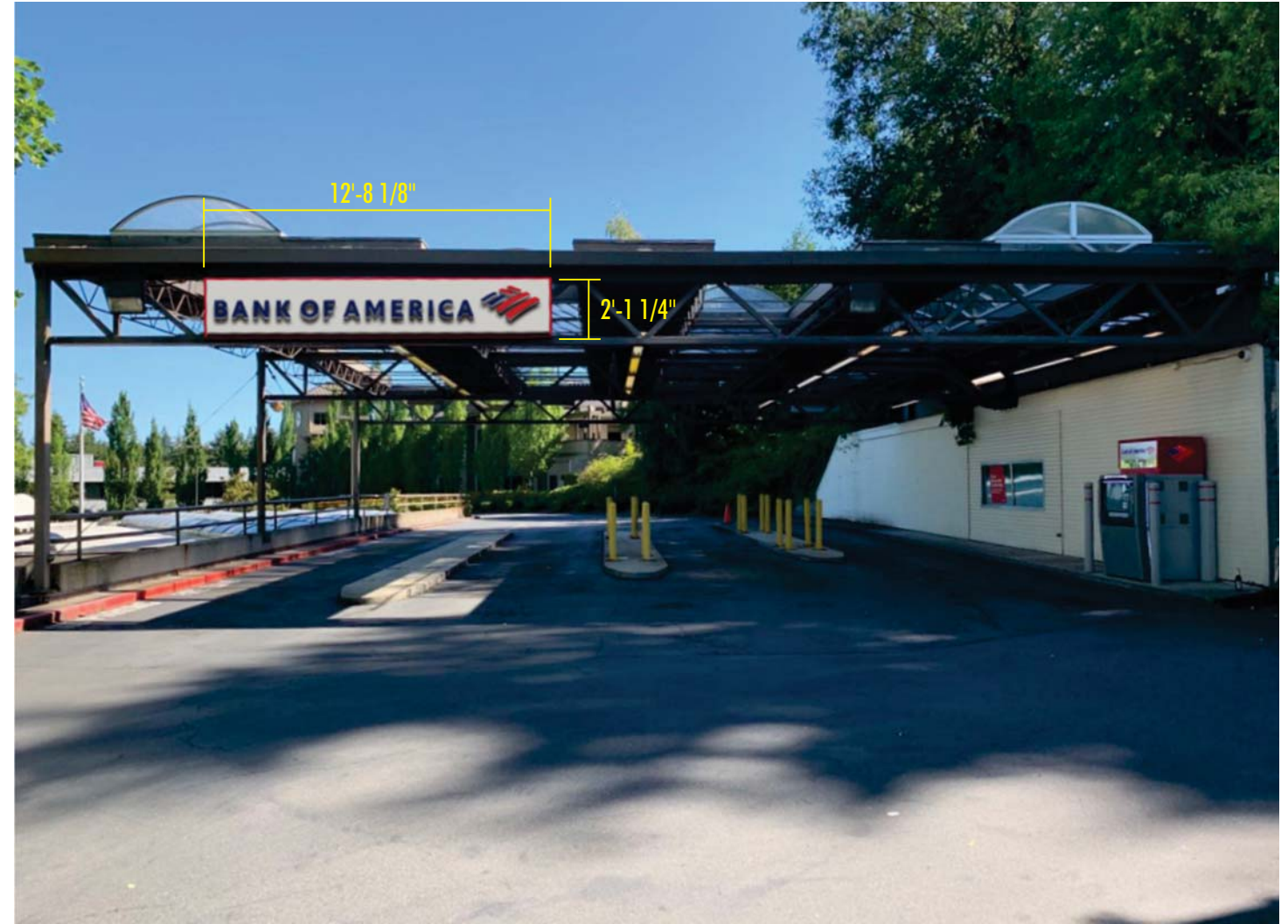
B2 PROPOSED SIGNAGE | CENTER VERTICALLY ON FASCIA IN SAME POSITION AS EXISTING SIGN 003 NOTE: POWER SUPPLIES TO BE HOUSED IN CUSTOM ALUMINUM RACEWAY MOUNTED TO BACK OF FASCIA (PAINT SATIN BLACK)
